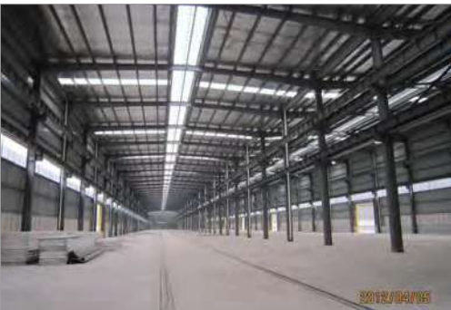
钢结构厂房 Steel structure workshop
