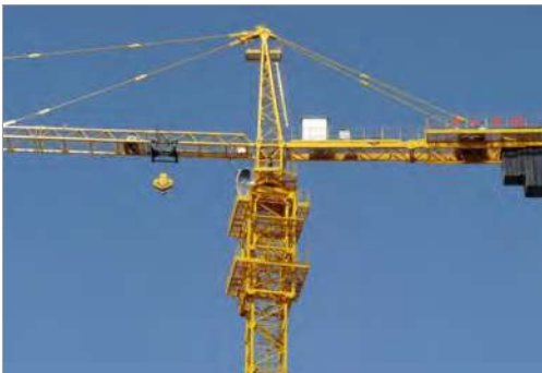
建筑塔吊 Tower crane
