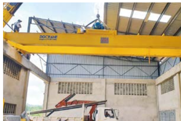
▲ LH20t Double Girder Overhead Crane in Kenya
