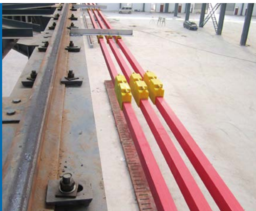
▲ Crane Rail & Bus Bar
