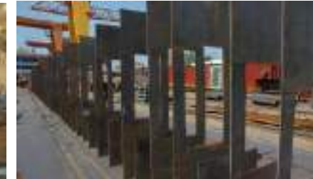
Tie-in and weld
